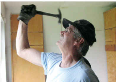
Ed Cale, an alumnus and parent, continues in the footsteps of Blue Mountain Academy's pioneering supporters as a volunteer in a recent renovation project.
