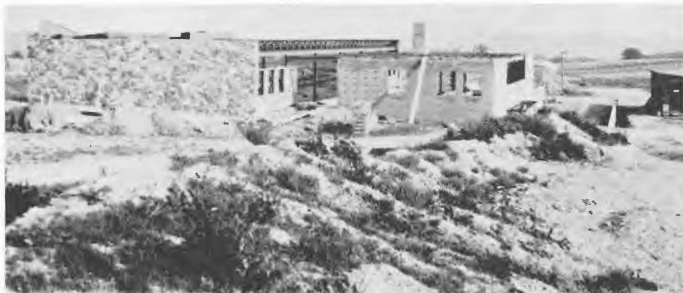
Rear of the Dining Hall, Showing the Kitchen
