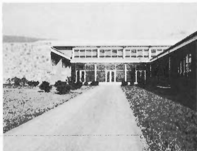
South entrance to Ad Building
