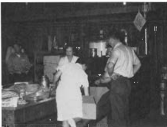
All the conveniences of a modern kitchen
