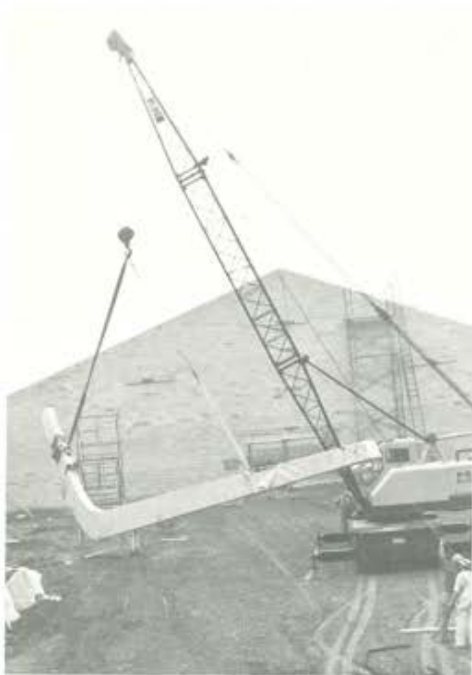
The first of 18-5000 lb Beams
