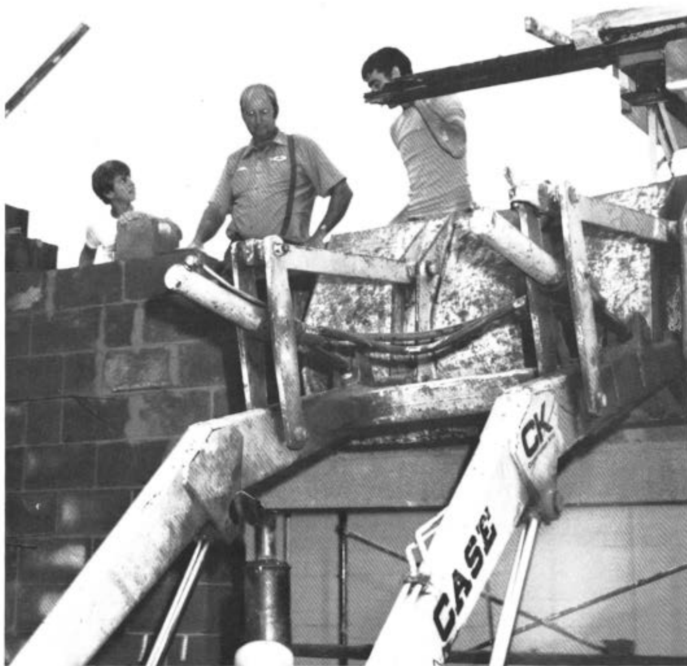
ABC UNDER CONSTRUCTION
